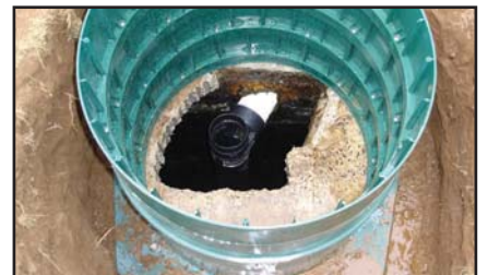
With risers installed
